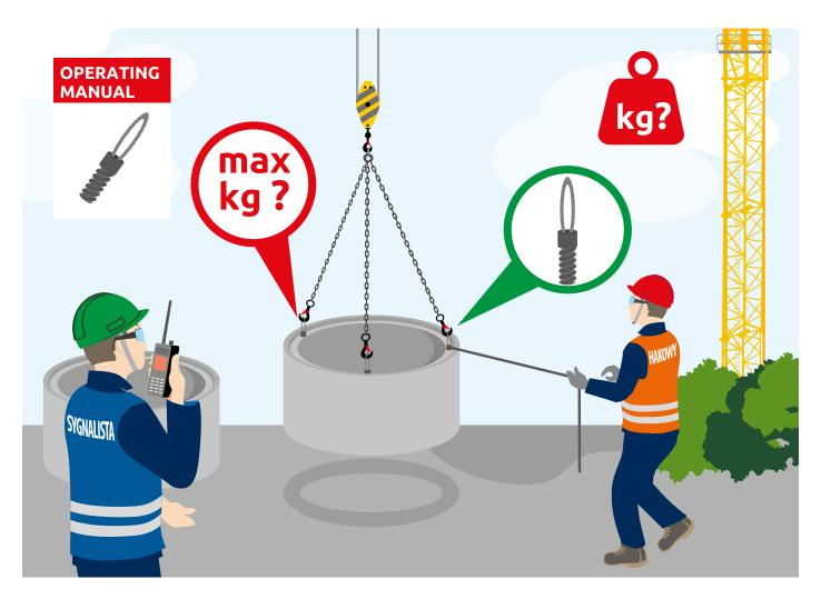
Rings should be transported and attached using clamps for rings in accordance with an operating manual of a manufacturer of the clamps and their working load limit.
