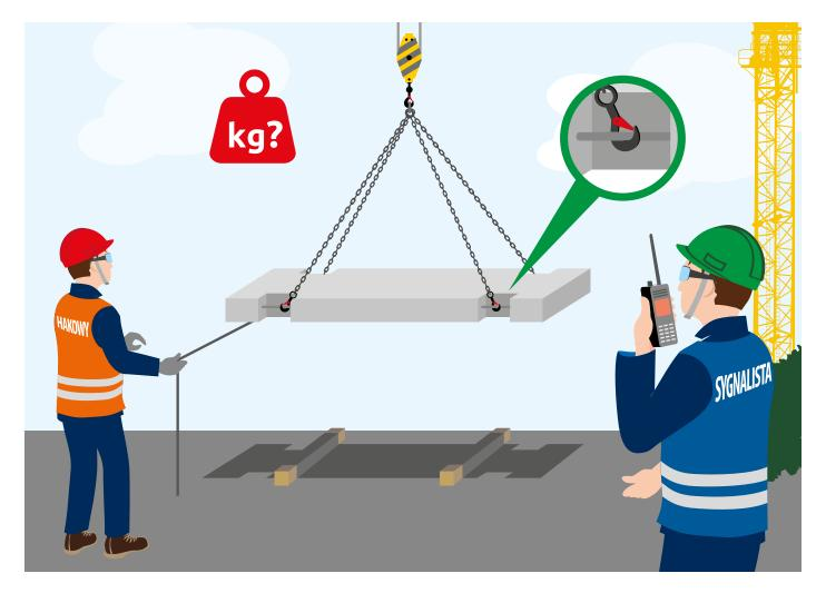
Road slabs with lugs should be transported using 4-leg chain slings.
